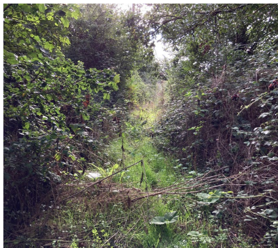
Existing FP200 where vegetation has grown over the designated route
