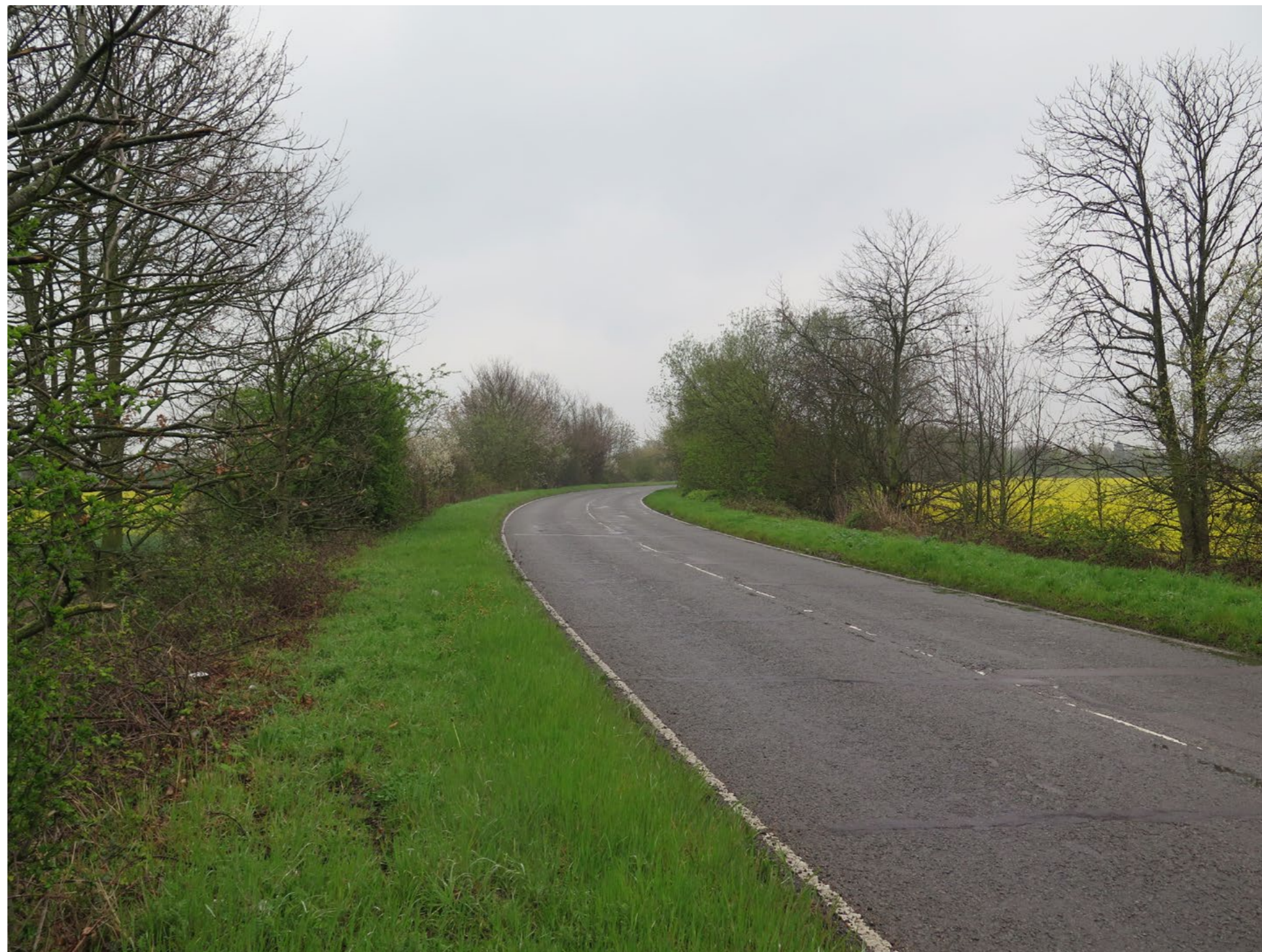
Existing Dennises Lane
