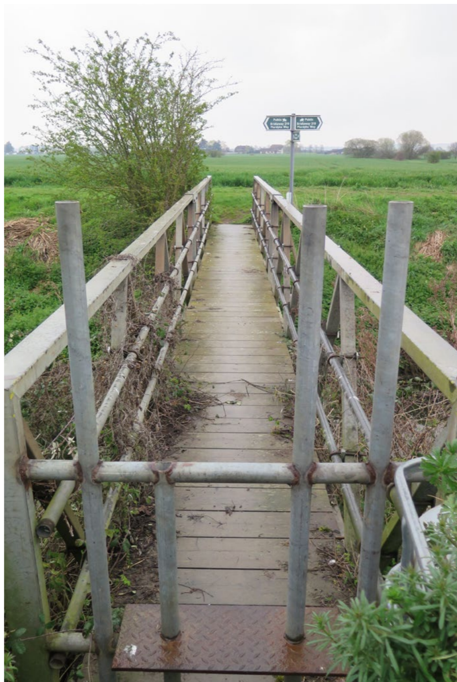
Existing FP136 bridge
