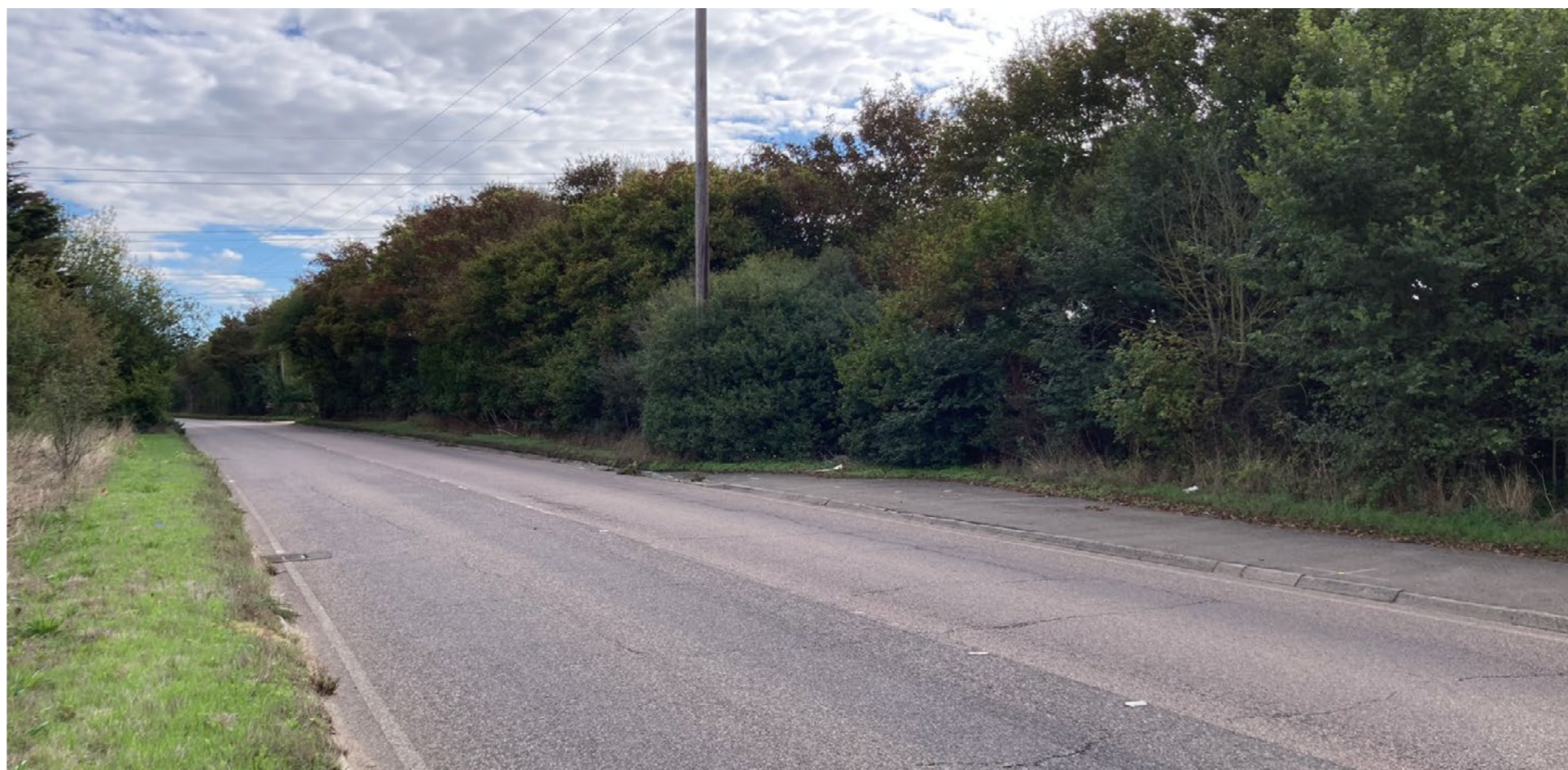
Existing shared pedestrian-cycle track along Stifford Clays Road, stopping abruptly with no further off-road provision
