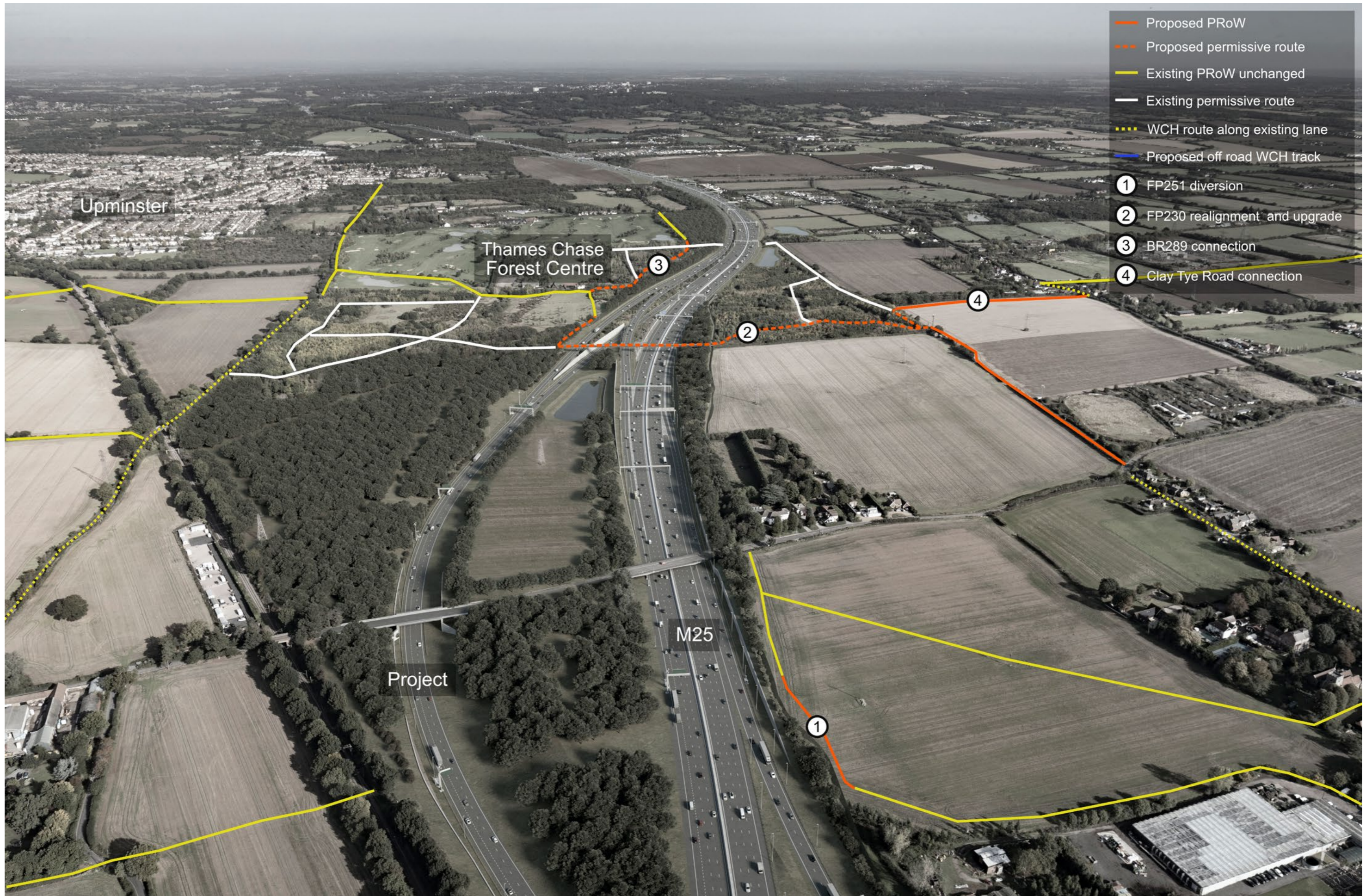
Aerial image showing WCH routes at the M25 Junction
